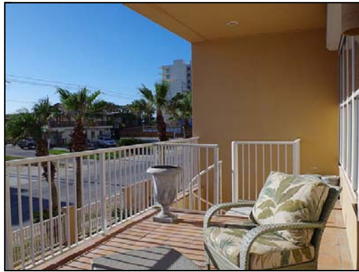
2nd floor balcony 2nd floor balcony is accessible from living area
