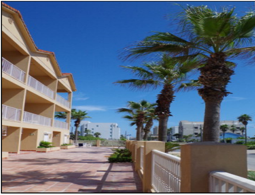
front of building
