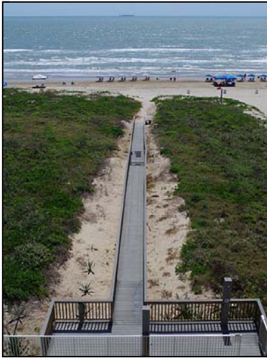
walkway to beach view of walkway to beach from unit 3301
