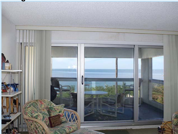
The living area has a floor-to-ceiling triple sliding door with impact-resistant glass.
