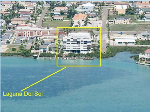
Laguna Del Sol is located directly on the bayfront.
