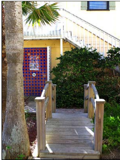
Courtyard Footbridge through courtyard.
