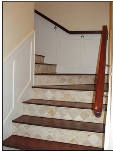
Stairs 2nd to 3rd
