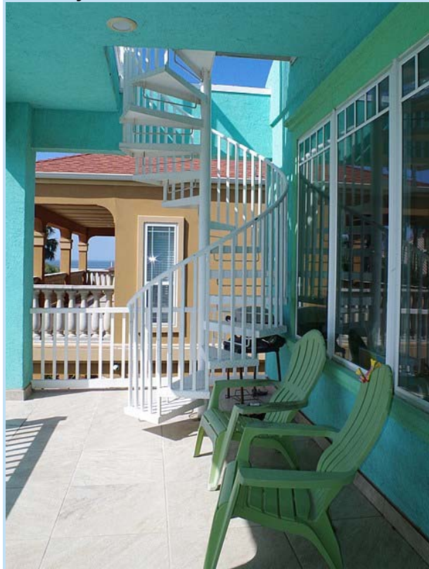
custom built spiral staircase to observation deck
