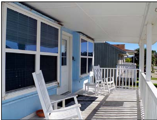
2nd floor deck
